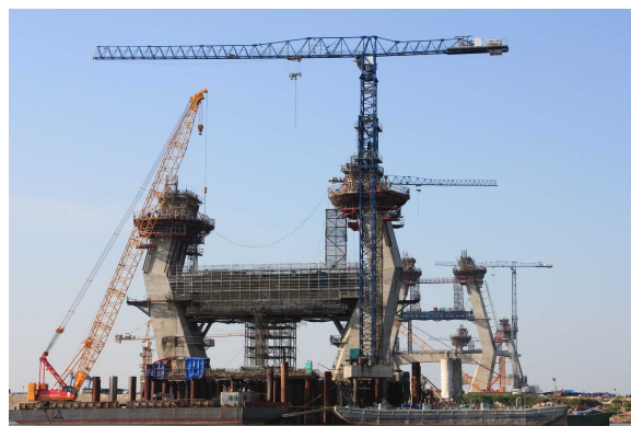
(Photo) Main tower construction with self-ascending/descending work platforms (Courtesy of Sumitomo Mitsui Construction)
