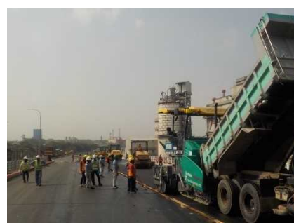
(Photo) PMB paving
