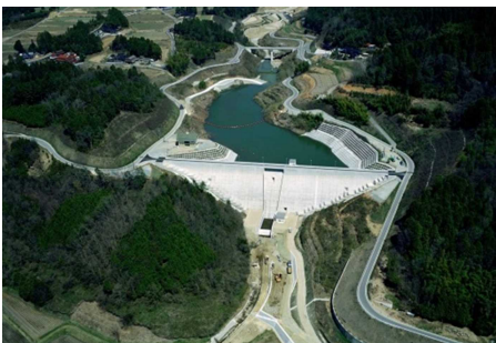
Construction of Dam
