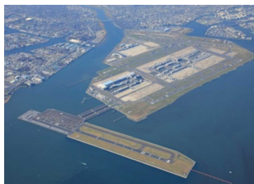
Tokyo International Airport (Haneda Airport) Runway D
