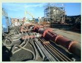
"Tornado Mixing Method", being one of the pipe-mixing solidification methods, produces and delivers solidification-treated soil with desired strength by adding a solidification agent to soft soil during the process of its pneumatic transportation and by mixing them with use of the plug flow. "Tornado Mixing Method" is remarkable in that it does not choose type of pneumatic transportation systems, enabling application to either seaborne reclamation works or shore-based reclamation works.
