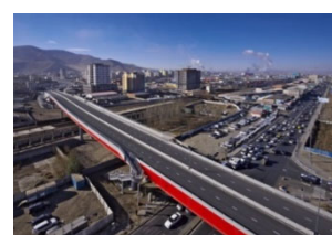
Railway Fly Over Bridge in Mongolia
