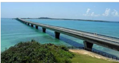
Ikema Bridge Prefecture : Okinawa Year of completion : 1992 Bridge type : PC continuous box girder Products : Viscous dampers with Al-Mg thermal spraying
