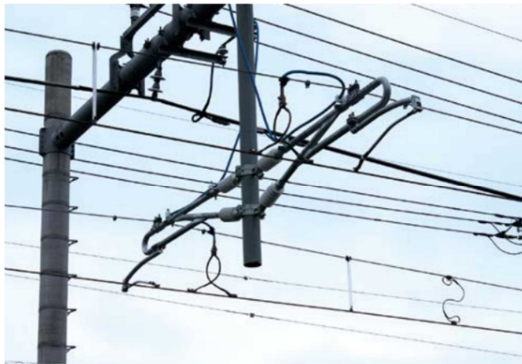
Hanger Ear Type B (Left), Type D (Right) Combination Example: Hanger Ear + Messenger wire protector
