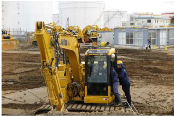
3 <Test Ride of ICT Construction Machine>
