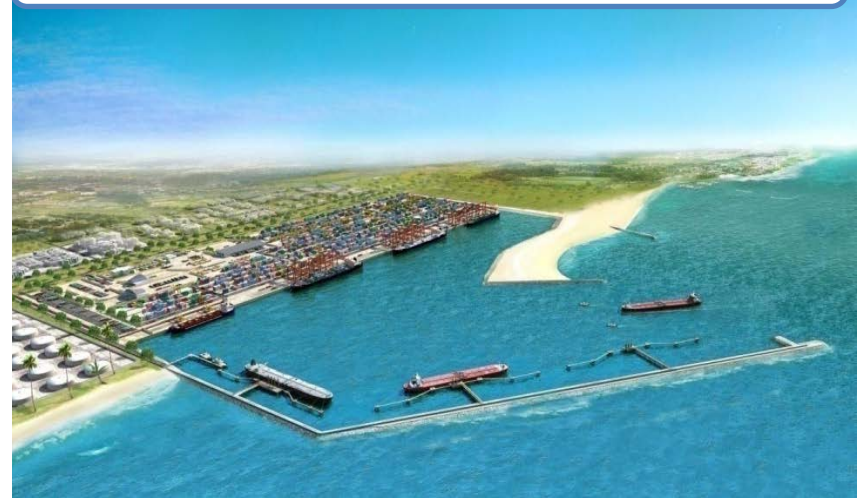
Lekki Port – Nigeria : $1.5B
